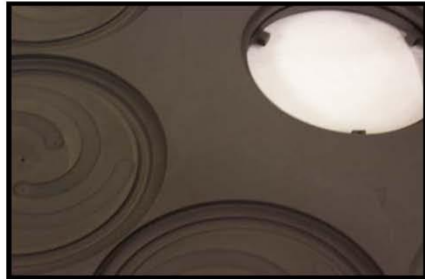
Cleaned using ThermaGas® process
